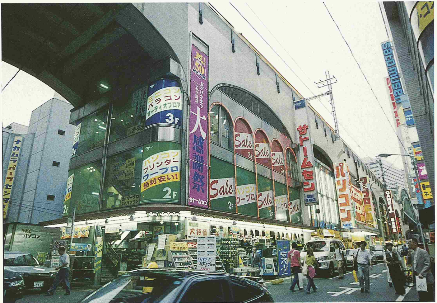
«Electric passage»; function: railway bridge + shopping arcade/ site: sotokanda, chiyoda-ku: In front of the west exit, Akihabara Station, Sobu Line – stacking and extension of the railway line and electric goods district – the railway tracks become a roof to 3 floors of electric goods shopping – 300 m length of shopping arcade – the scale of the frontage of each shop divides this section of railway into smaller and smaller proportions
