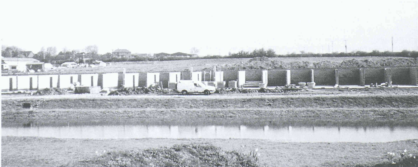
Hockerton Housing Project in der Grafschaft Nottinghamshire
