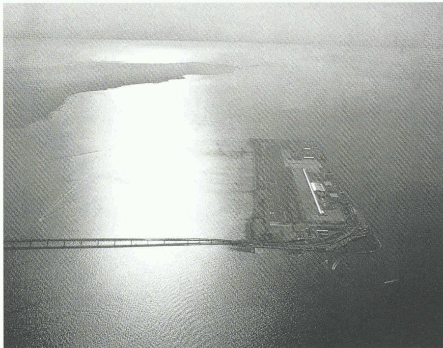
The Kansai Air Terminal, Osaka Bay, Japan (Photo: Sky Front)
