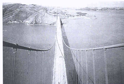
Golden Gate Bridge
