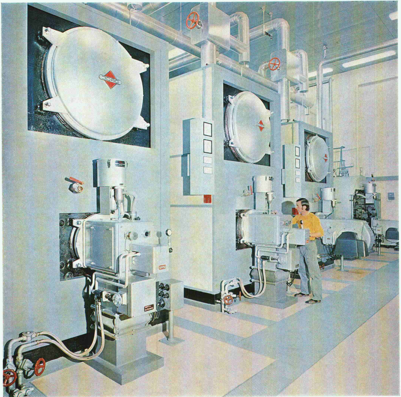
Bürgerspital Solothurn, Heisswasseranlage, 180 °C, 13 atü: 2 Kessel 4 Mio Kcal/h, 1 Kessel 3 Mio Kcal/h, 1 Kessel 2 t HDD, 13 atü
