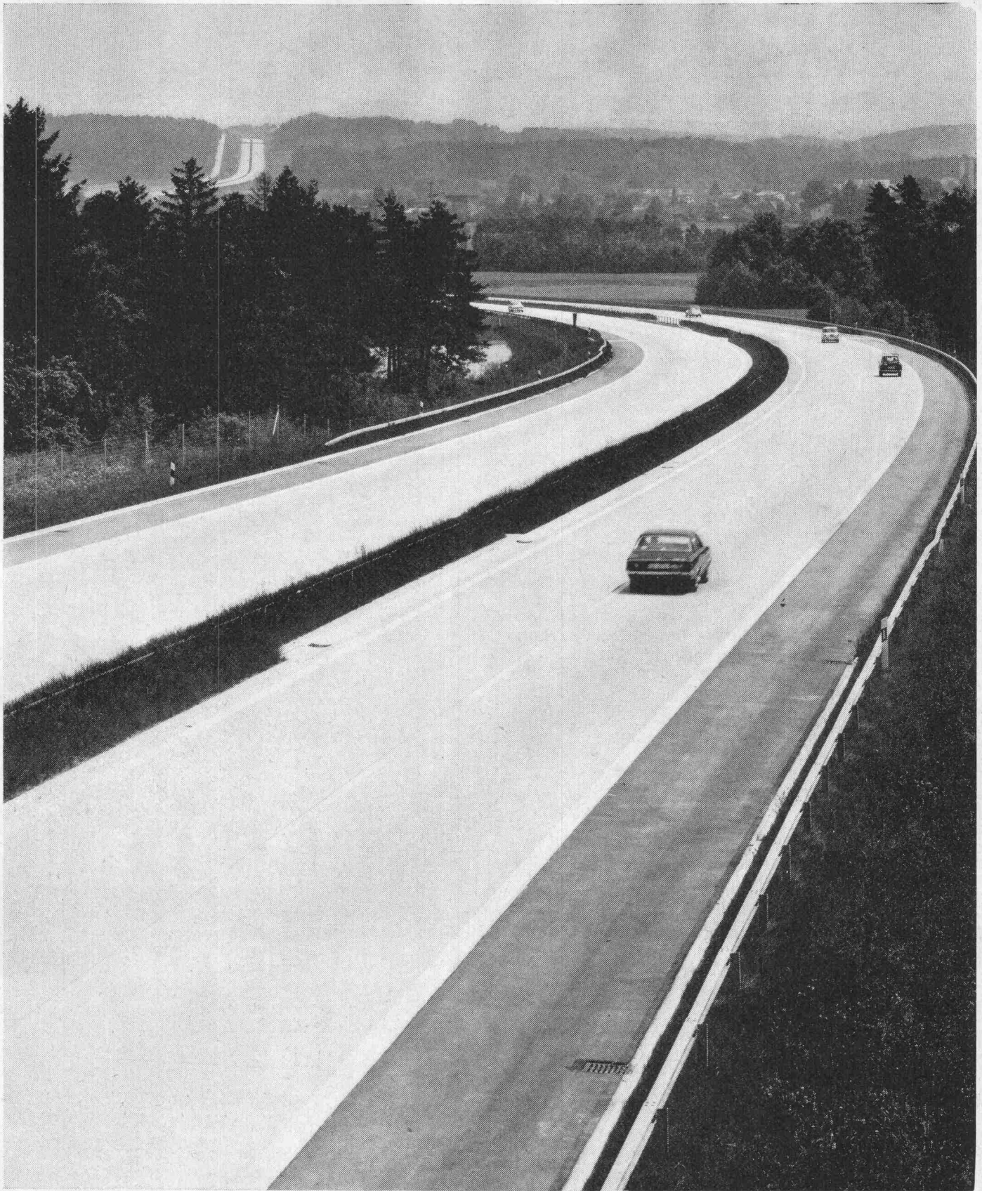
Nationalstrasse N 1 Wil—St. Gallen, Betonbelag
