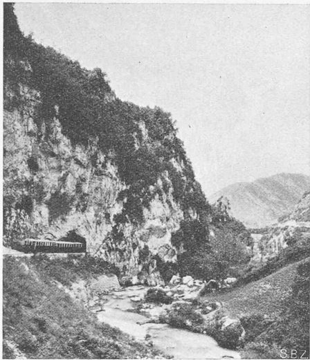
Abb. 9. Oberes Portal des Tunnels Balza tagliata I (122 m lang). Km. 35,2 (talwärts).
