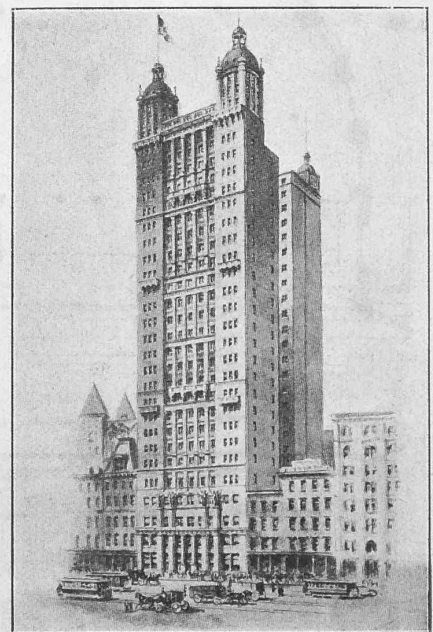
Abb. 17. New-York. — Park Row Office Building.
