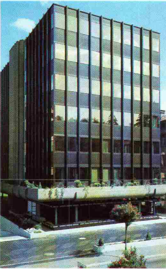
Palazzo Benzug, CH-Lugano, 1977 INFRASTOP-Gold 40/26 Arch. L. Doninelli, Bellinzona
