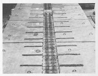
Fig. 12. Arrangement of the connection reinforcement for the TTp-shoulder support. In practice the connections above the beam between the slab units are instead made in form of projecting stirrups
