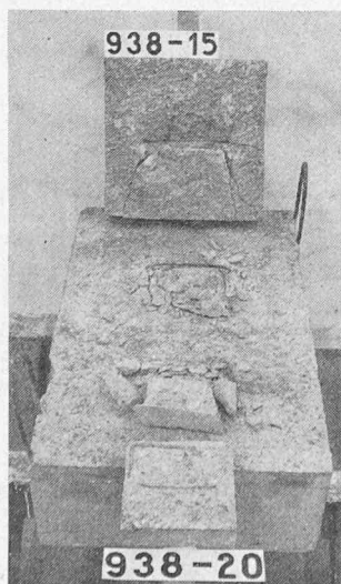
Fig. 10. Types of anchor rupture of stirrups cast into a thin concrete topping. Note the difference in type of rupture for smaller (15×15 cm 2 ) and larger (30×30 cm 2 ) surfaces. When size was (61.5×61.5 cm 2 ) the rupture was a pure tension cone around the stirrup
