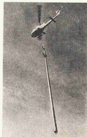
Transport eines 26-m-Mastes
