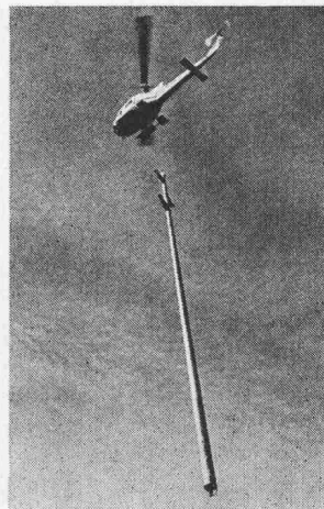
Transport eines 26-m-Mastes
