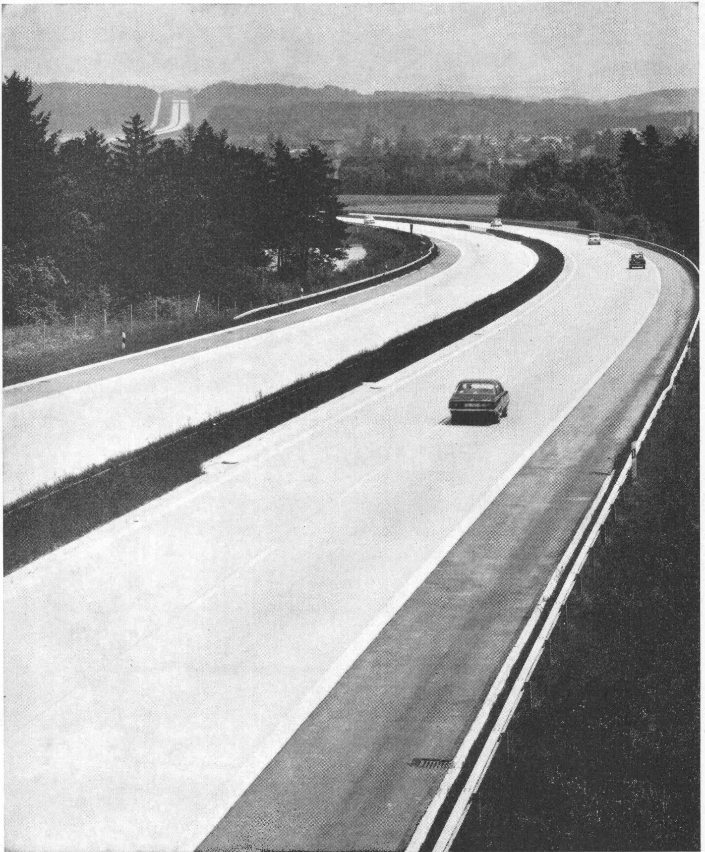
Nationalstrasse N 1 Wil—St. Gallen, Betonbelag
