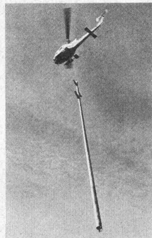
Transport eines 26-m-Mastes
