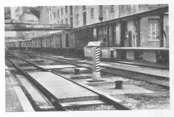
Abb. 6. Waggonwaage System Wirth in Basel
