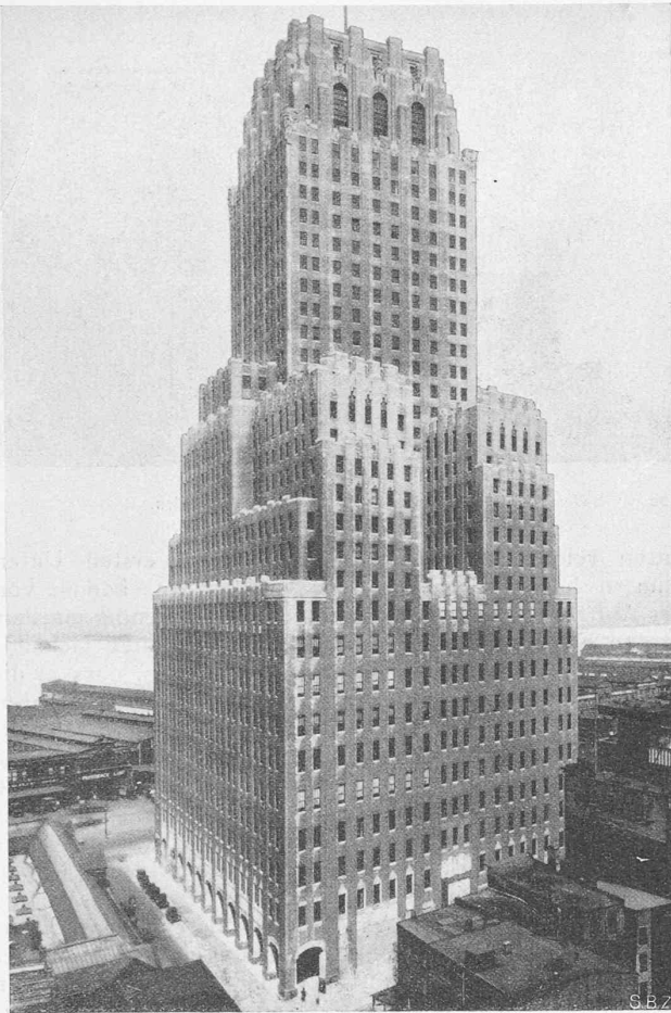
Abb. 7. New York Telephon Building am Hudson River.
