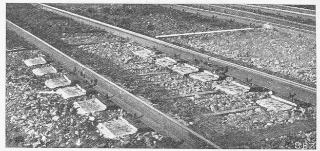
Abb. 1. Eisenbeton-Schwellen System Emperger.
