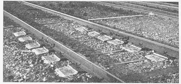
Abb. 1. Eisenbeton-Schwellen System Emperger.
