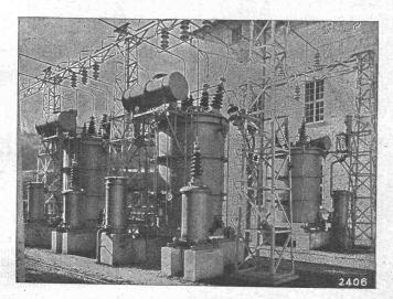
FORCES MOTRICES GRISONNES, STATION TRANSFORMATRICE EN PLEIN AIR DE KUBLIS, 3 TRANSFORMATEURS MONOPHASÉS 4500 kVA, 10800 A 67600 VOLTS, 162/3 PÉR/SEC.
