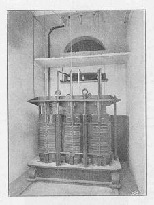
Abb. 12. Transformator, A, 1900 KVA., 3750/27000 V.
