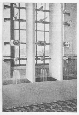
Abb. 58. Wasserstrahlerder 50 000 Volt. Station Piattamala.
