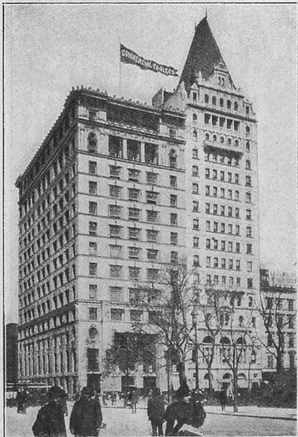
Abb. 13. New-York. — Postal Telegraph Building.
