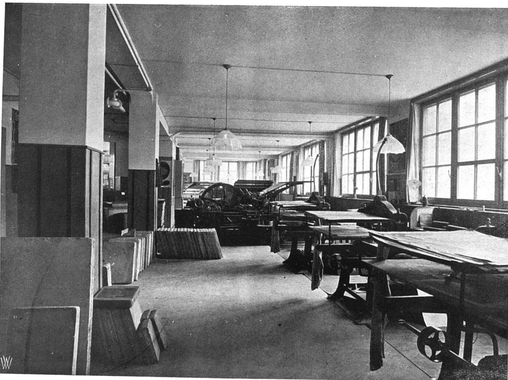
Blick in den Maschinenaal II
