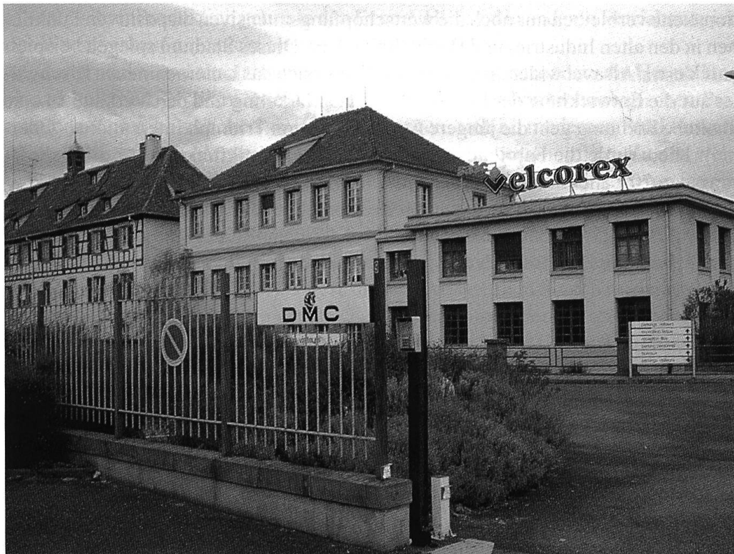
Abb. 6 Weberei SAIC Velcorex in Colmar.
