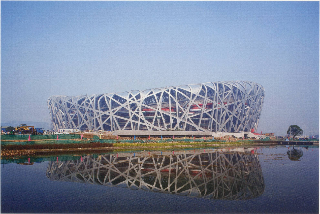
National Stadium Beijing, under construction, 2007.
