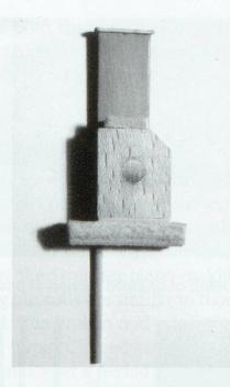
Figure 5: Detail of a replaced lead weight in a bass damper.
