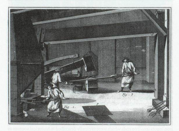
Figure 4. Straining the iron into rods (from Diderot, 1758).
