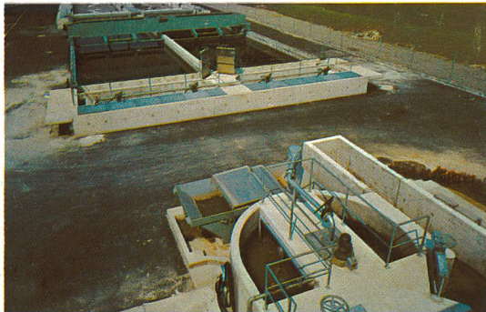
Rundsandfang, System Pista ARA Pfungen
