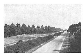
Fig. 5. Freeway with continuous shoulder and heavy planting near an intersection. A strip of grass between the median hedge and the roadway disguises the asymmetry of the road half.
