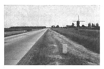
Fig. 7. Unplanted freeway in keeping with the structure of the landscape. Only one roadway has been built. The space on the right is intended for the second roadway.
