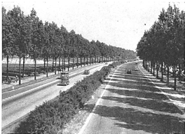
Fig. 1. Freeway with double rows of trees along the cycle paths. The way on the right was recently transformed into a three-lane road to increase capacity. On the wide median a freely growing hedge.
