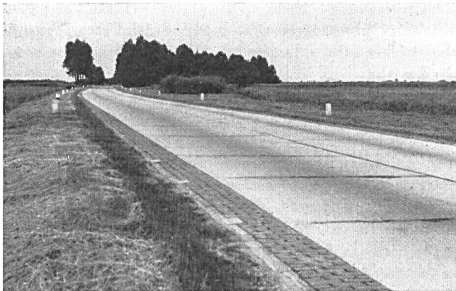
Fig. 4. Freeway of which only one of the two lanes has been built. The planting on the unused part of the road lot gives a pleasant accent to the open landscape. The space for the future second lane is on the left. The absence of median planting favourably affects the space picture. The parking lane has not yet been built, which promotes the symmetry of the road.
