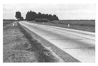
Fig. 4. Freeway of which only one of the two lanes has been built. The planting on the unused part of the road lot gives a pleasant accent to the open landscape. The space for the future second lane is on the left. The absence of median planting favourably affects the space picture. The parking lane has not yet been built, which promotes the symmetry of the road.
