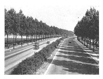
Fig. 1. Freeway with double rows of trees along the cycle paths. The way on the right was recently transformed into a three-lane road to increase capacity. On the wide median a freely growing hedge.
