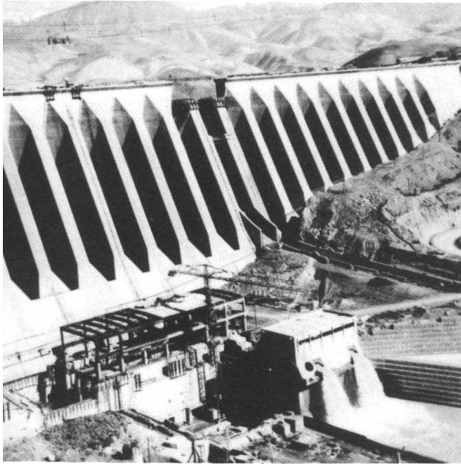
Barrage de Latiyan, Iran
