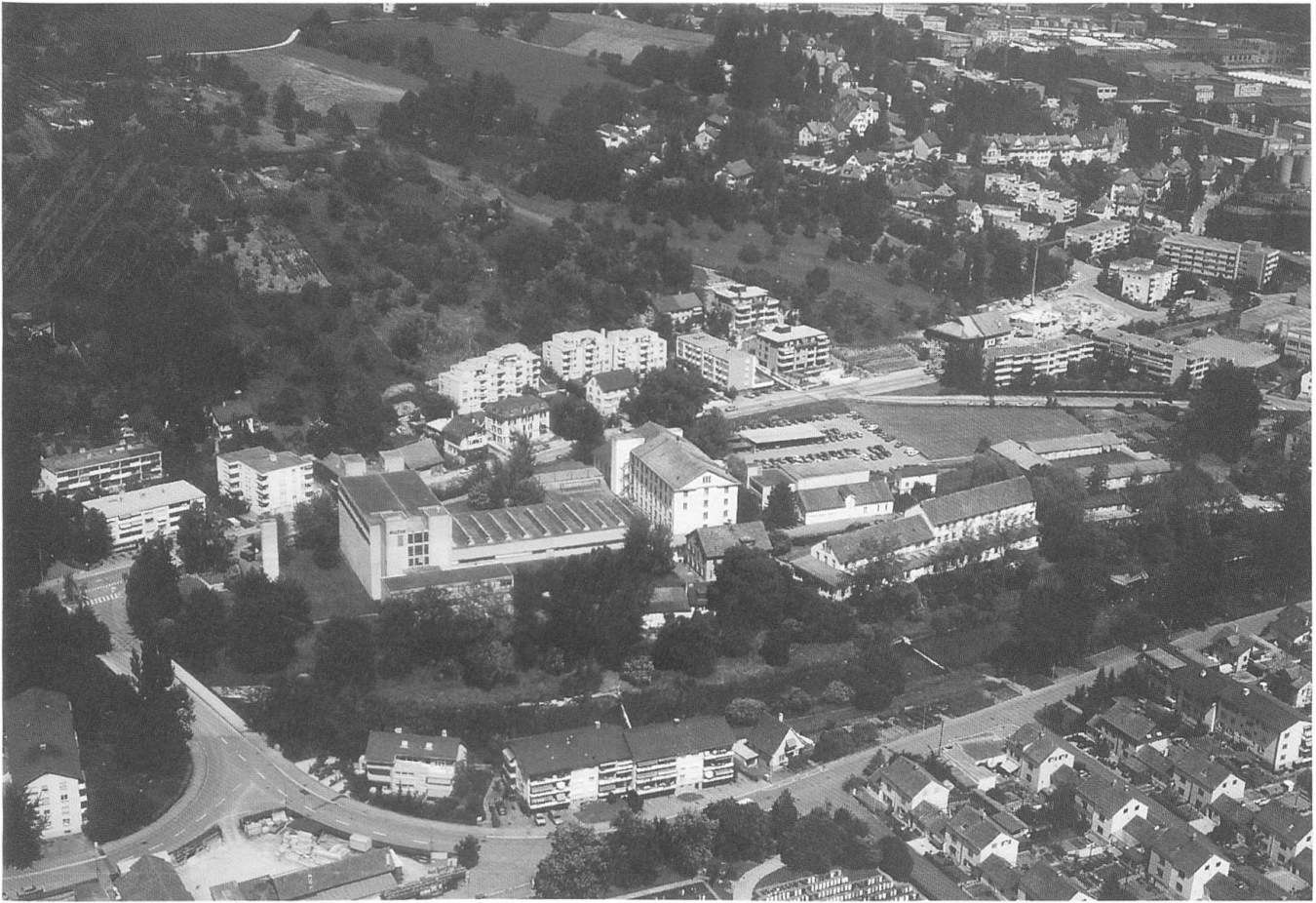
Research and development centre in Nieder-töss
