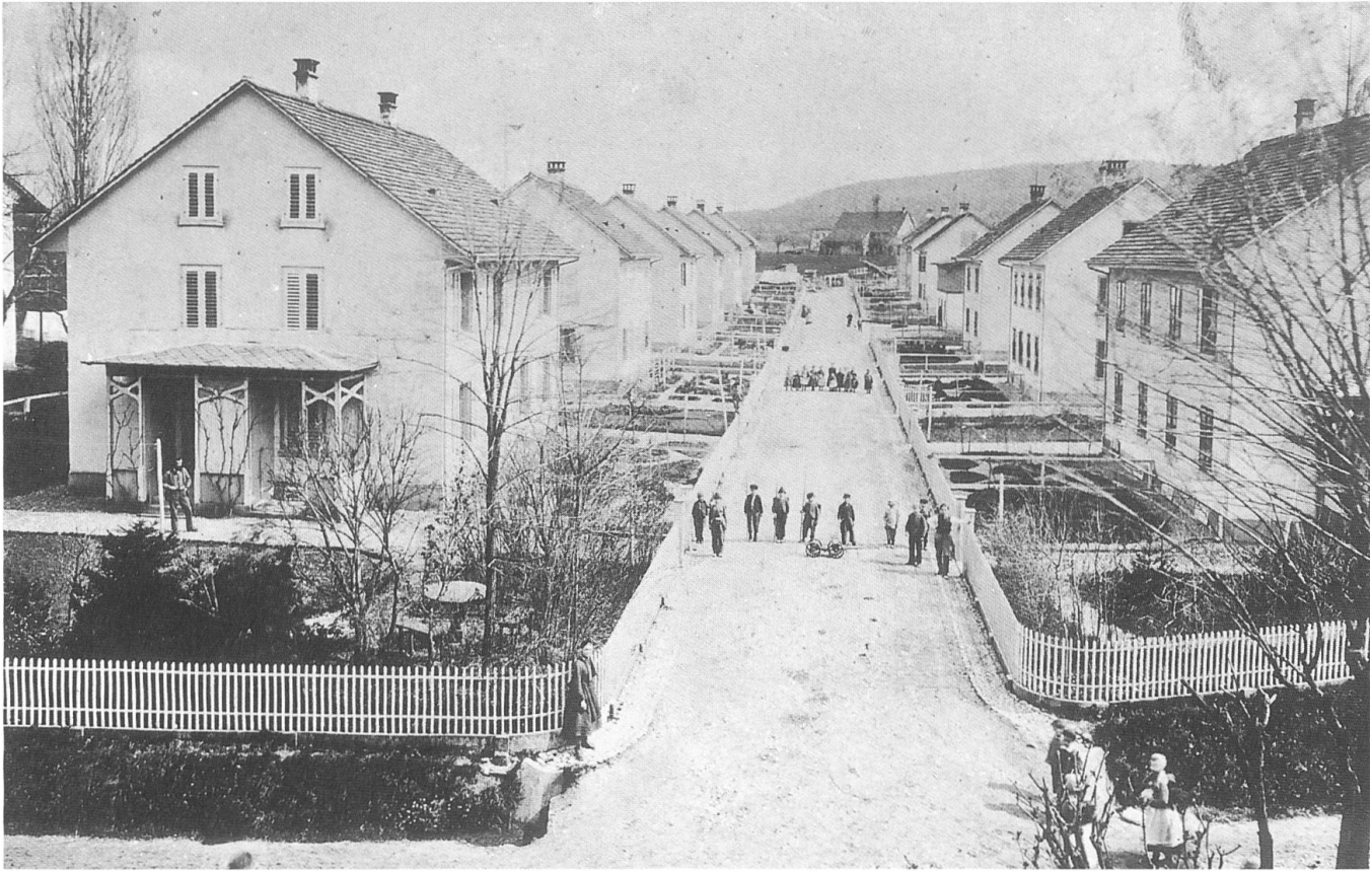
Workers' housing estate in Töss, under construction from 1865; shown above on a photograph ca. 1870, below after the latest renovation
