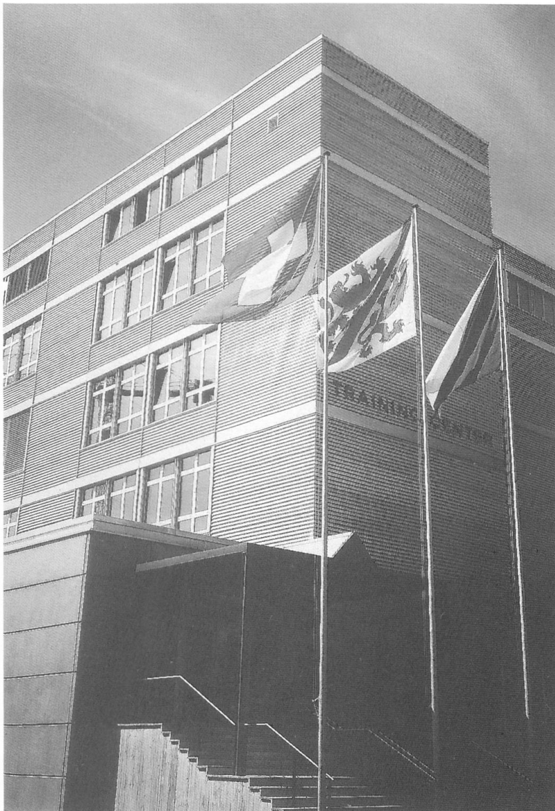
The training centre, built in 1990 and used mainly for customer training
