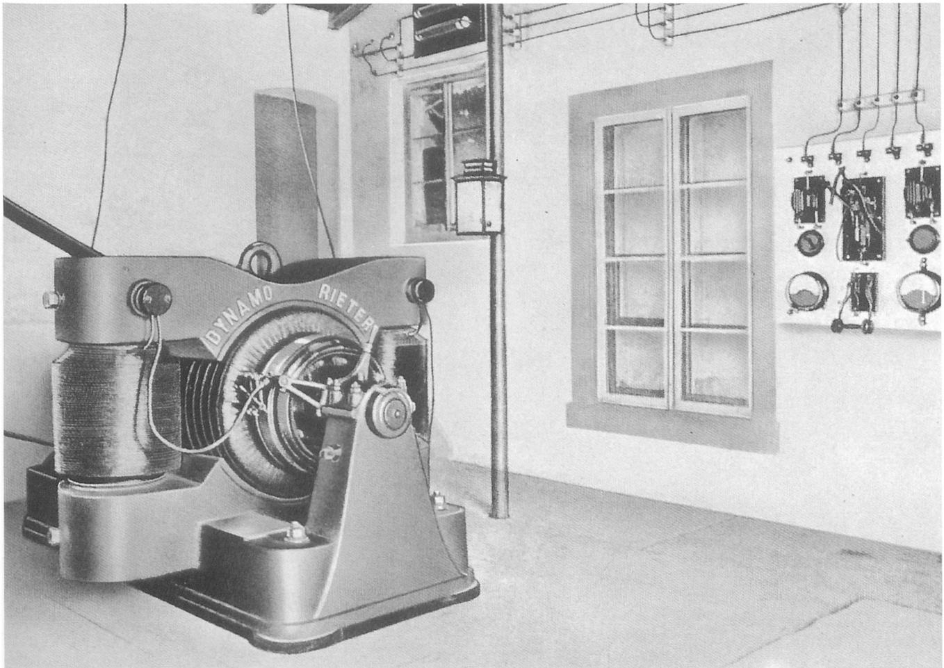
*Generator with an output of 100 kW, 1892*
