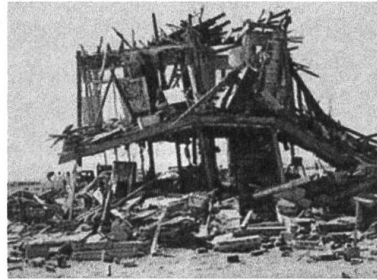
15., 16. Wood frame house before and after a nuclear explosion, Nevada Test Site. Samuel Glasstone, editor, The Effects of Nuclear Weapons , prepared by the United States Atomic Energy Commission, 1962
