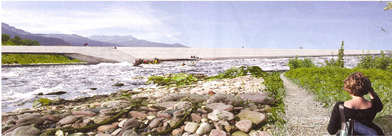
Ansichten einzelner Plattformen View of the various platforms
