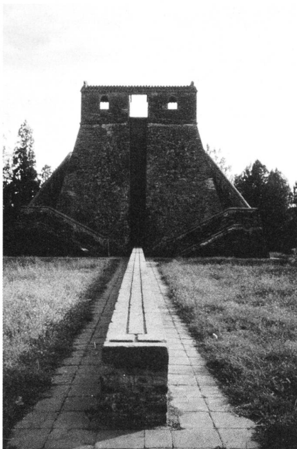
Fig. 1. Huge gnomon at Gaocheng, Henan province, built in A.D. 1276 by Guo Shoujing. The shadow of the vertical gnomon, 9.8 m in height, was projected on a horizontal scale, 31.5 m in length; this scale was placed due north of the tower. Pinhole imaging was used to accurately define the shadow edge. This allowed accurate calendar determination, particularly of the solstices and equinoxes, and also the days on which festivals or ceremonies, as decreed by the emperor, should be held. Photograph courtesy of ARNOLD VON ROTZ.
