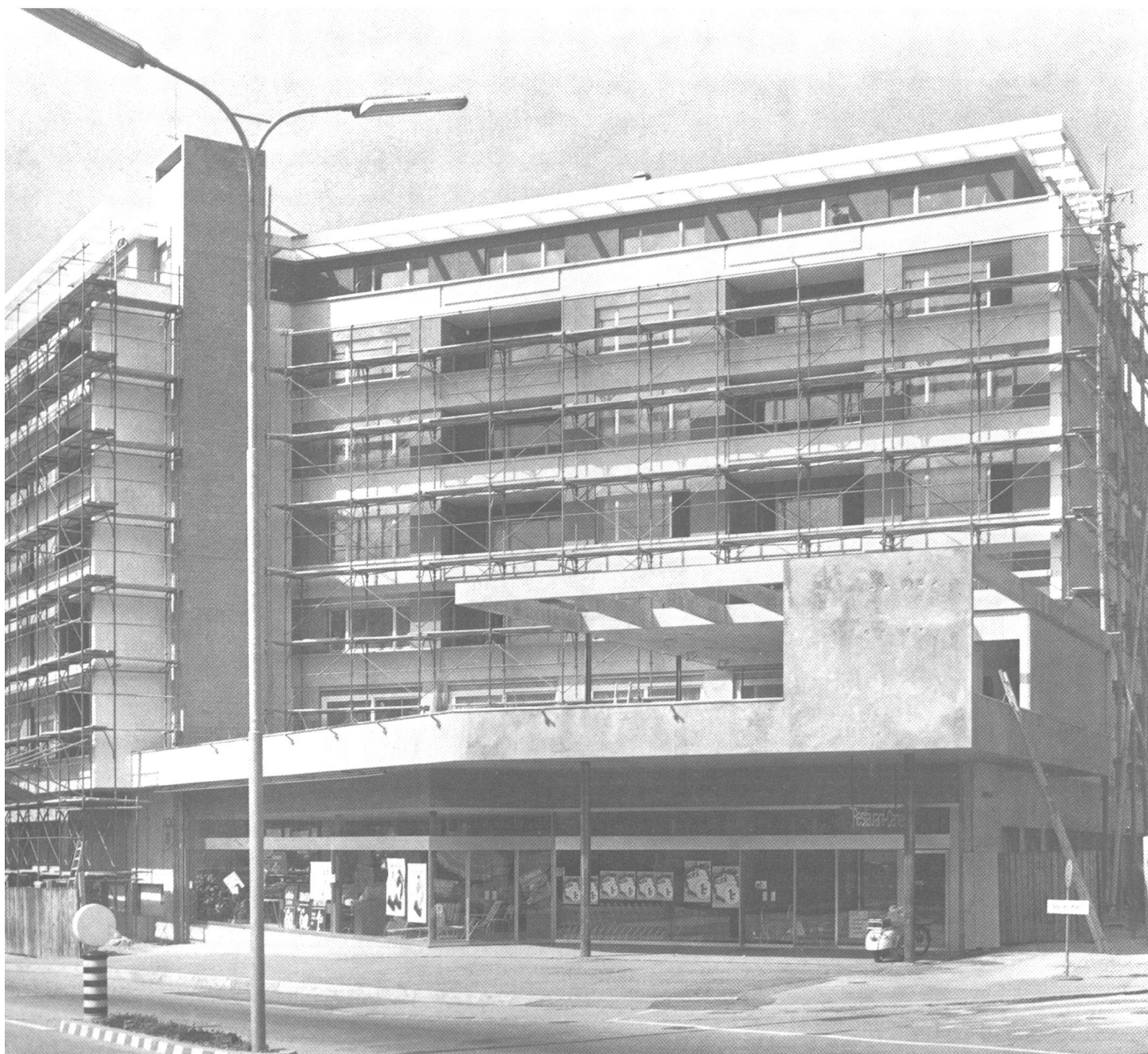
Coop-Center am Bifangplatz in Olten
