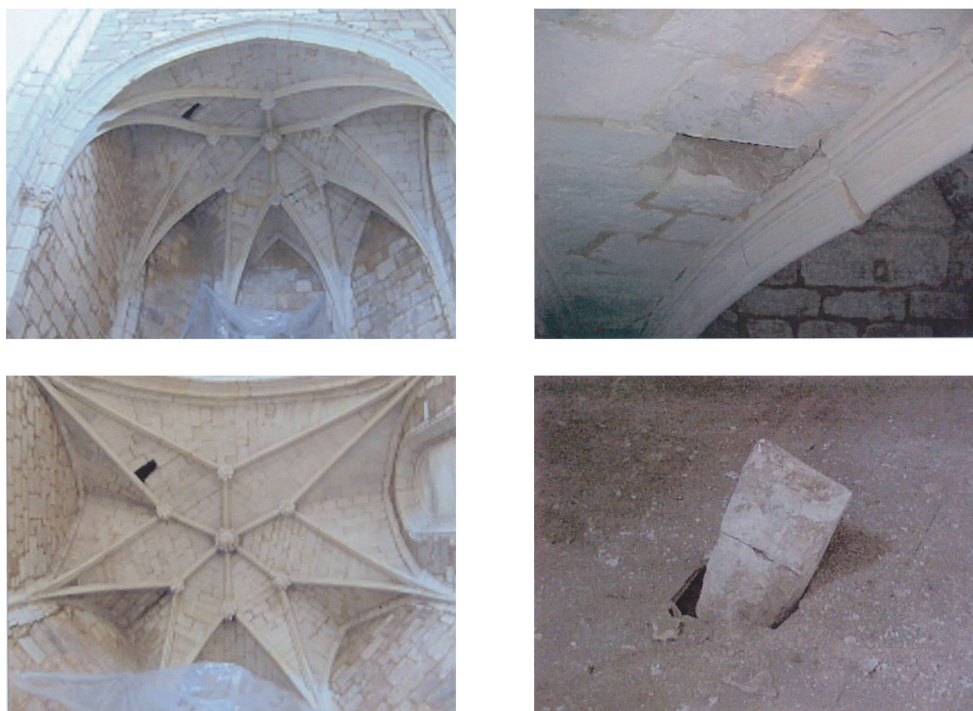
1 A stone falls down from the web of a gothic vault in a parish church in Burgos (Photo S. Huerta Fernández).
