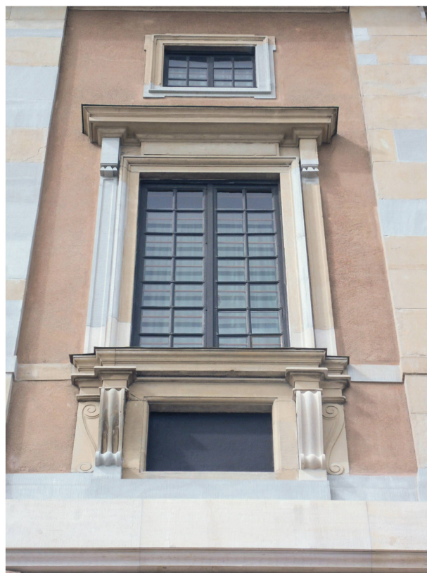
3 The façade after stone replacement. Old Gotland stones are a dark yellowish grey, new Gotland or Rorschacher stones are a blueish grey and new Obernkirchener stones are a light yellowish grey. Whether the colour differences are acceptable or not is a matter of ideology and taste (Photo A. Heymowski).
