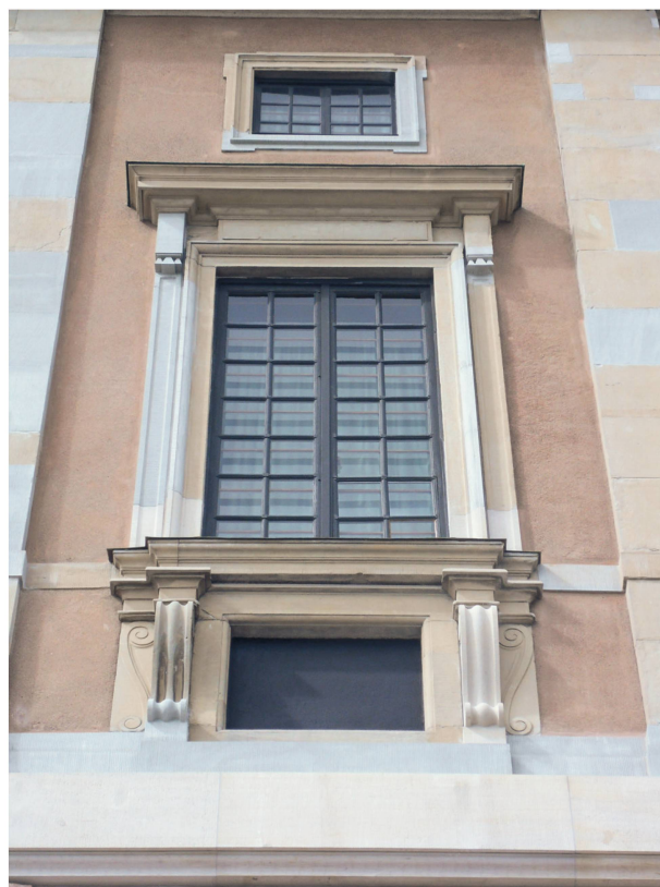
3 The façade after stone replacement. Old Gotland stones are a dark yellowish grey, new Gotland or Roschacher stones are a blueish grey and new Obernkirchener stones are a light yellowish grey. Whether the colour differences are acceptable or not is a matter of ideology and taste (Photo A. Heymowski).
