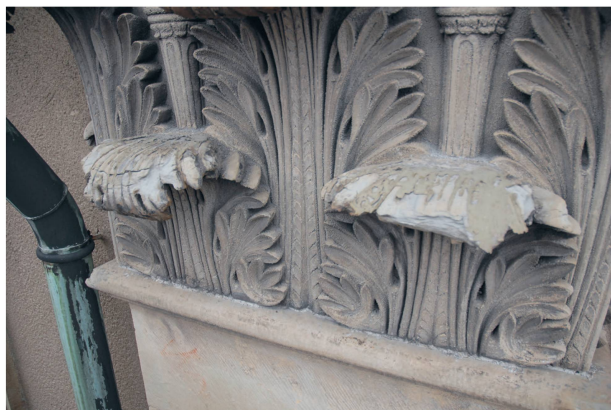
2 A Corinthian capital, bearing traces of a vain attempt around 1970 to preserve its protruding acanthus leaves by coating them with fibreglass reinforced plastics (Photo Mikael Traung).
