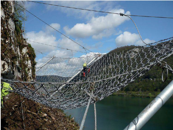
Figure 11. –Filet de protection de 3000 kJ (Nantua); photo BG / Hugues Foltzer.
