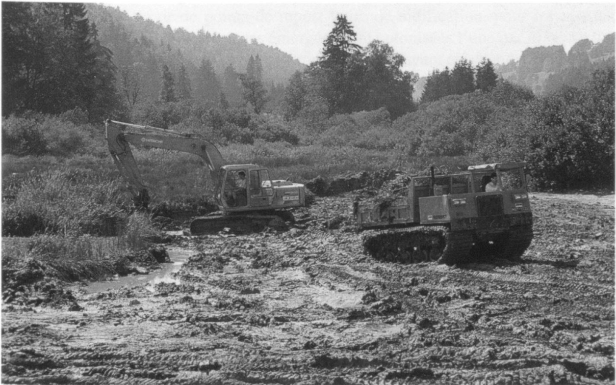
Figure 8: Travaux de creusage (Photo Fr. Gfeller, 10.8.1995).
