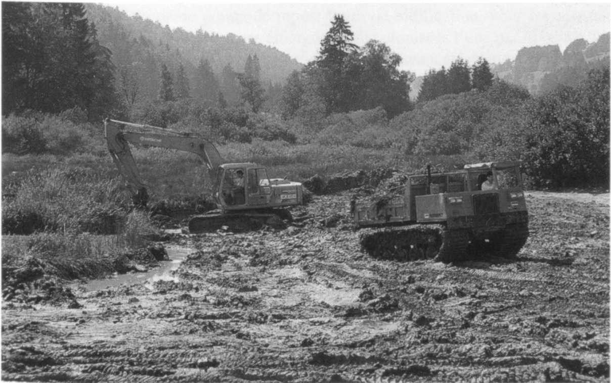
Figure 8: Travaux de creusage (Photo Fr. Gfeller, 10.8.1995).
