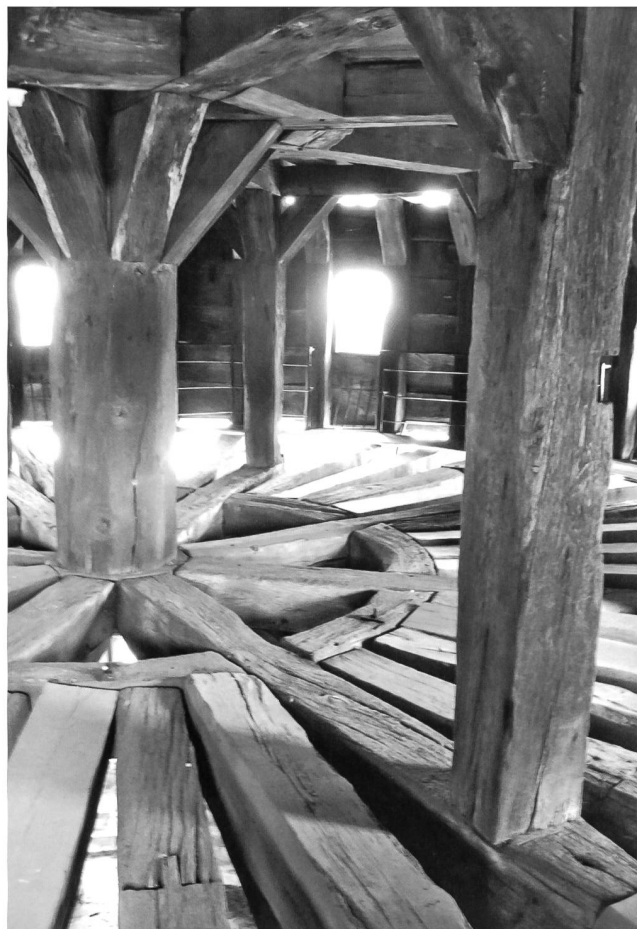
6: Laval, Dep. Mayenne (F). Innenansicht des Hurdengeschosses.
