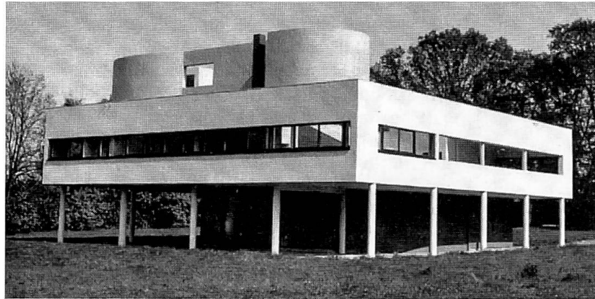
Abb. 3. Le Corbusier, Villa Savoye (1927–30) in Poissy. (Aus: Le Corbusier – Architect of the Century , Arts Council of Great Britain, 1987. Foto Fondation Le Corbusier, Paris)
