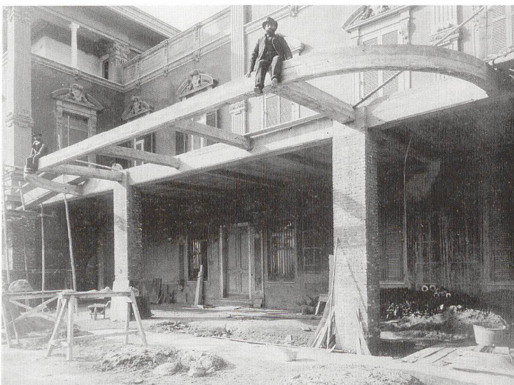
Quarto, Villa Quartara, 1905–06, Auskrragung in Eisenbeton System Hennebique. (Repro, S.172)
