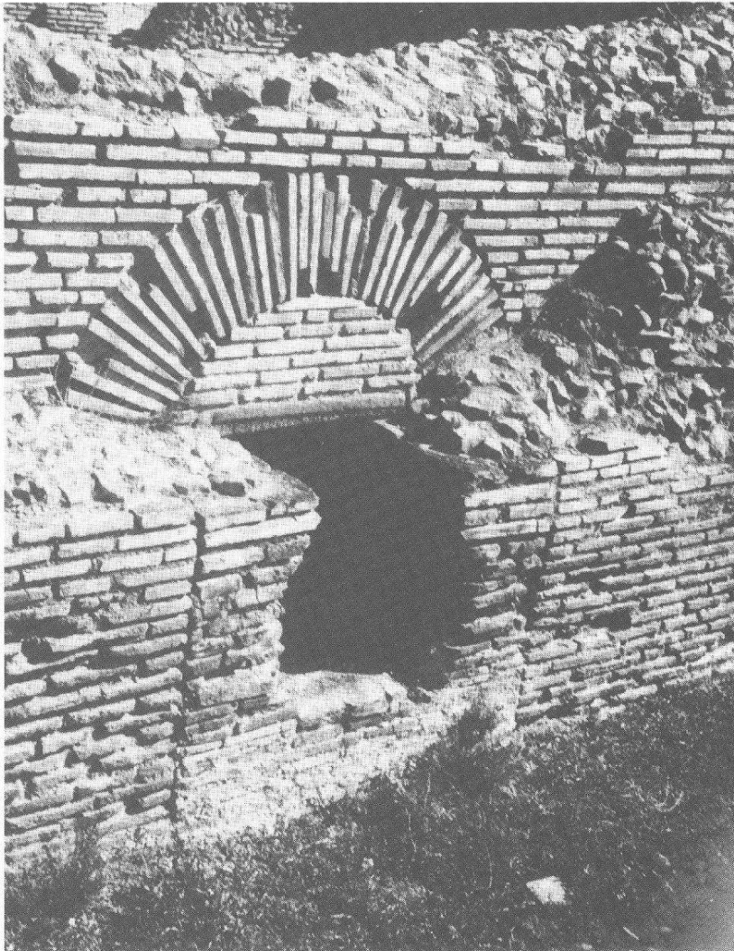
Abb. 2 Timgad, Praefurnium in den grossen Nordthermen.
