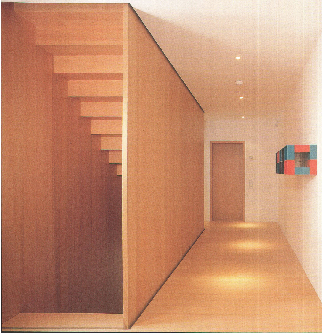
<Free-standing staircase made of boards of four centimetre thick Douglas fir and held together by stair treads of the same thickness.
