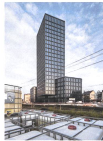
Grosspeter-Tower, Basel Burckhardt + Partner, Basel
