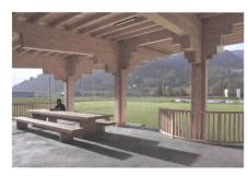
Massive Balken tragen das Dach. | Massive beams carry the roof.
