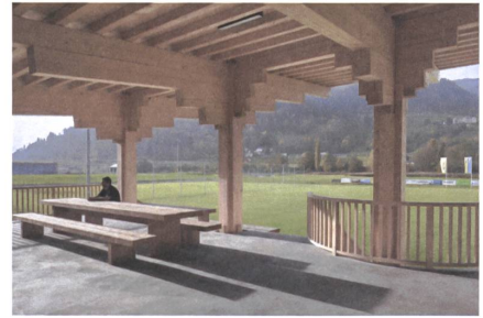
Massive Balken tragen das Dach. | Massive beams carry the roof.
