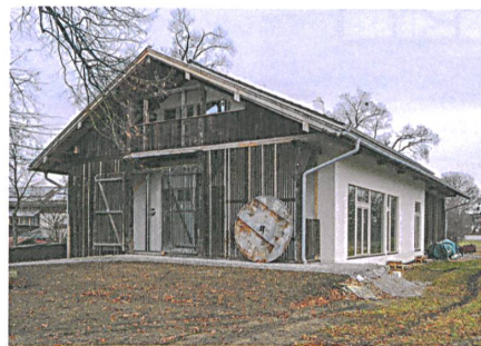
29 Die Torfremise am neuen Ort. | A new location for the shed.
