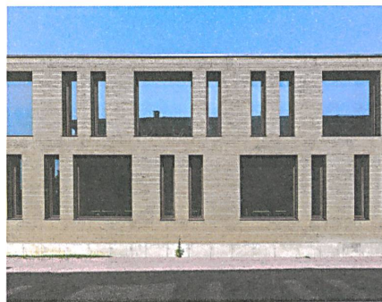
16 In den Mauern aus Stampflehm steckt kaum graue Energie. | Hardly any grey energy is used inside the rammed clay walls.
