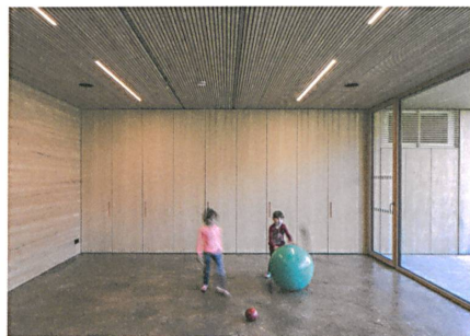
Böden aus Stampflehm. | Floors made of rammed clay.
